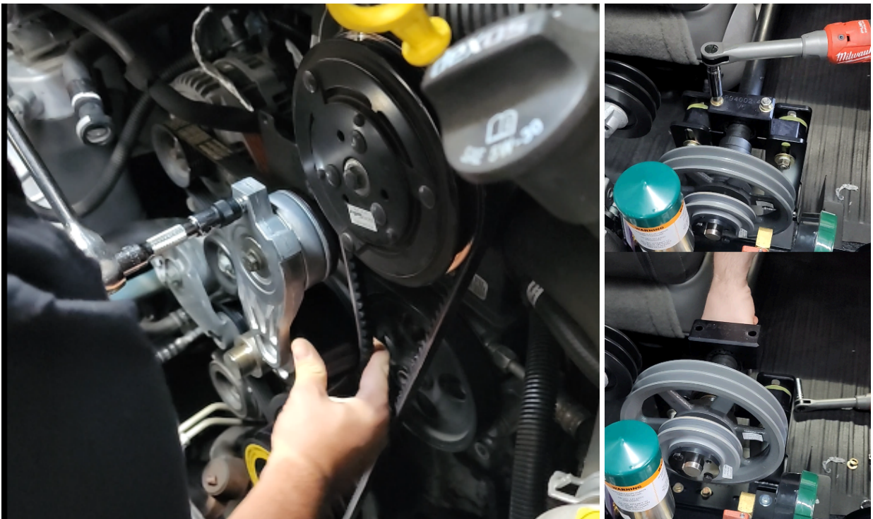
Cooling Fan removal is not required but removed for picture clarity.
